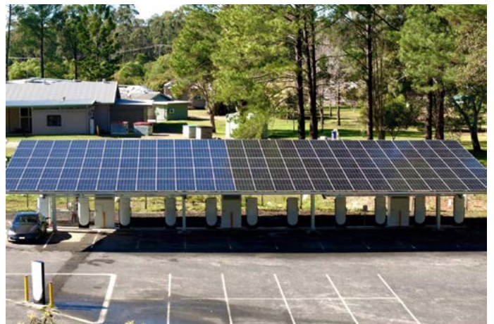
Top: The 12 bay Tesla Supercharger in the back car park. Eleven bays under the massive awning topped with solar panels. Note the stand alone bay designed for EVs with caravans /trailers in the left of the photo.
