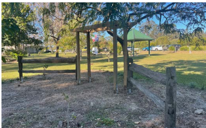
The two-rail slab and post fences were common on New Italy properties. The Antoniulli fence, once at the front of the Museum site, was removed as it became fragile and the highway upgrade progressed. Some of the fence has been repurposed to form the wedding bower in the Park of Peace.
