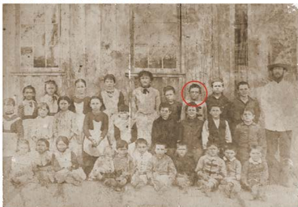
The first school building was made of slabs with battens on the cracks. Messieur Jean Le Cheminant, a French linguist who also spoke Italian, was appointed as the first teacher at the New Italy School in 1885.
